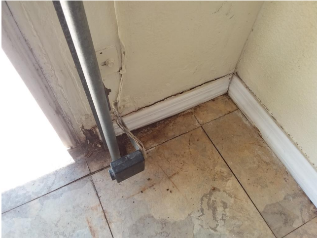
Wood decay (garage base boards)
