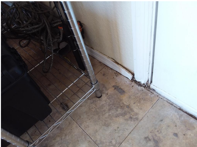
Wood decay (garage base boards)
