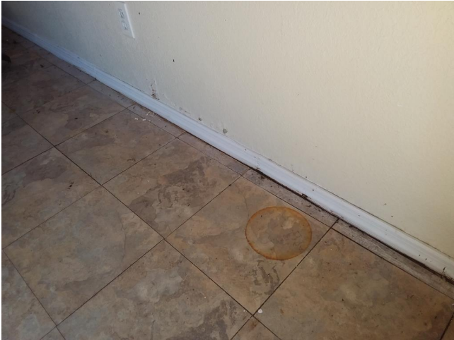
Wood decay (garage base boards)
